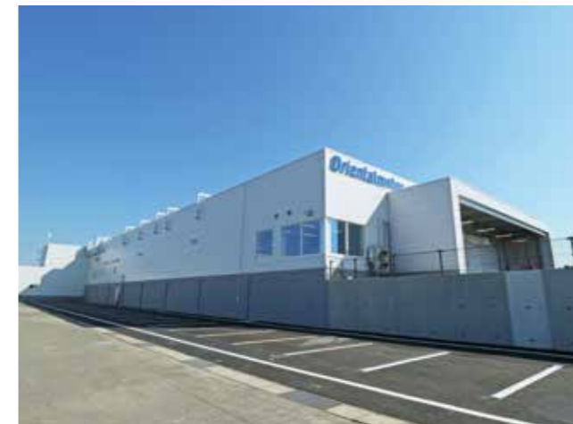
Plant building with a fill at Noshiro Oriental Motor
