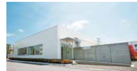
Reliability Testing Laboratory
