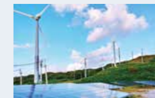
Solar Power Generation / Wind Turbine Generation
